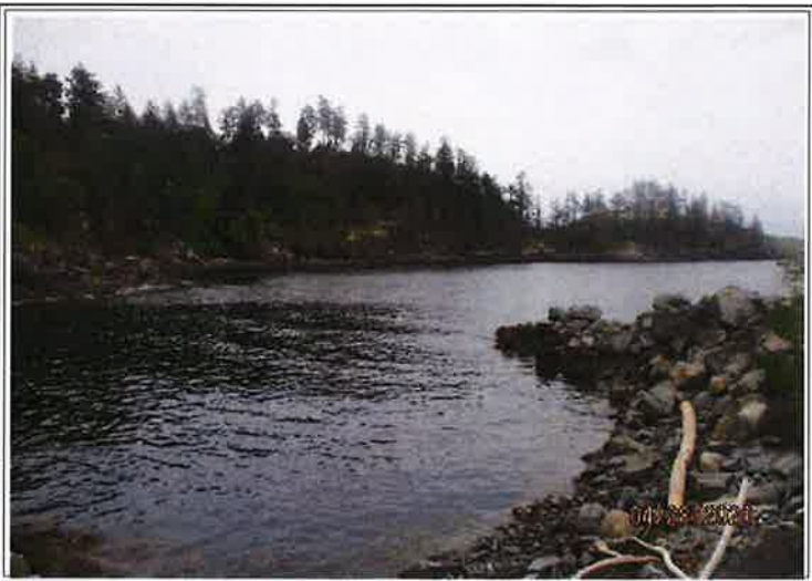
waterfront and breakwater
